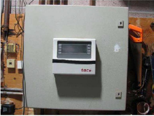
BMS Panel with Display Terminal
